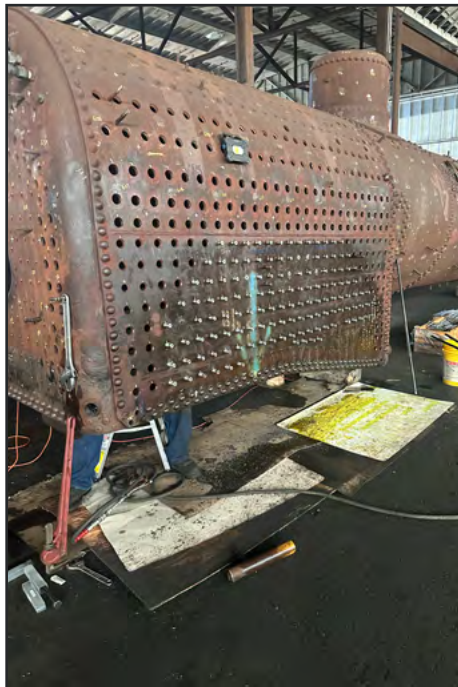
Alan Siegwarth photograph End of weekend photograph with the stays installed on the sidesheet.
