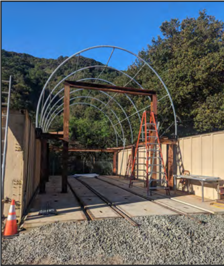
Stephen Barkkarie photograph Brightside M 601 repair enclosure framework.
