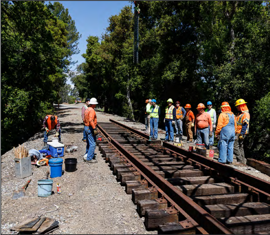
Building East crew lining panel.
