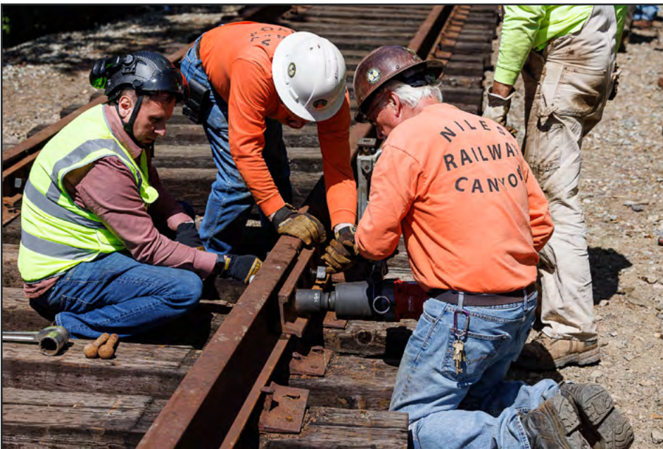
Pat Stratton using impact wrench to tighten track bolts.
