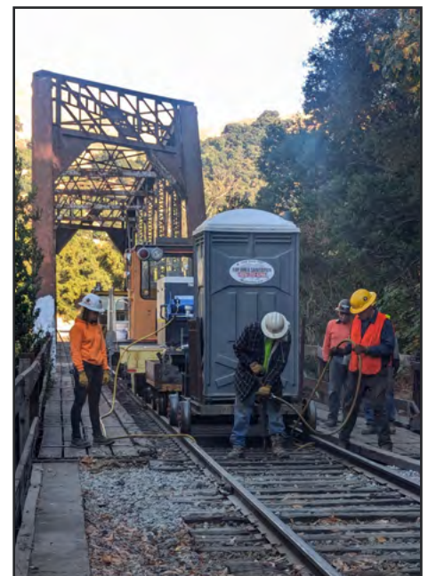
Stephen Barkkarie photograph Pneumatic hand tamping of first tie on approach.
