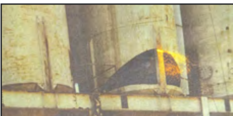
Mark Whitman cutting a slice so we can pull down a tippel cylinder. This was not an easy job.
