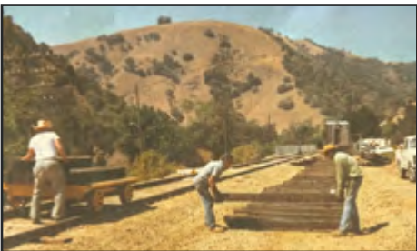
Track crew starting to extend siding at Brightside.
