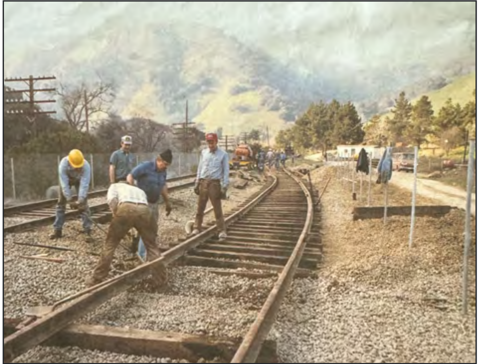
Track crew building what would become the passing siding at Brightside.
