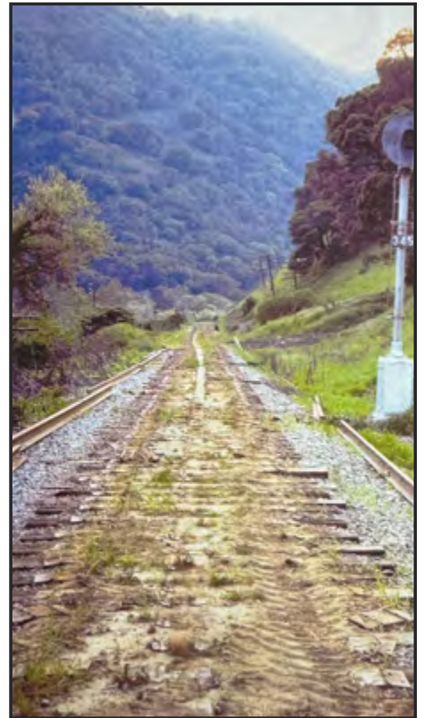
The S.P. took the rail and tie plates for a new passing siding in Arizona. We held onto the ties.
