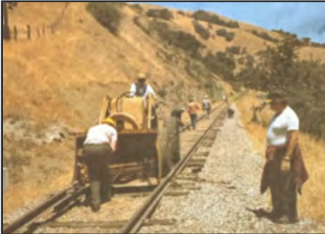
Track being replaced on the ties that remained after S.P. Departure.
