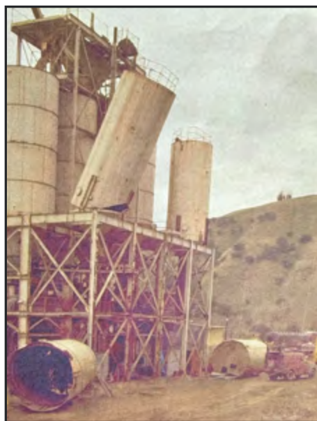
"Hit it!" Boom truck pulls a cylinder off the tippel foundation.
