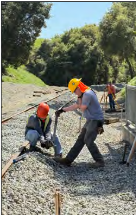
The "A" team setting top-of-rail stakes at Castlewood Bridge, April 5, 2025.
