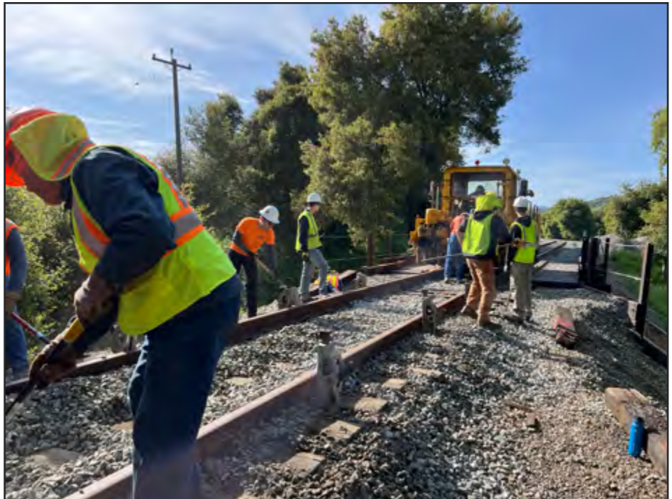
Raising and tamping track just east of Happy Valley Road bridge. April 5, 2025.
