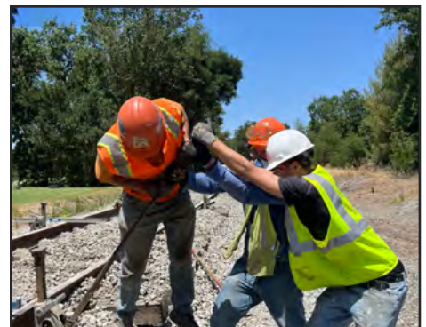
Track and ballast weigh a lot and it takes a lot of muscle to raise track. Mike Pechner photograph
