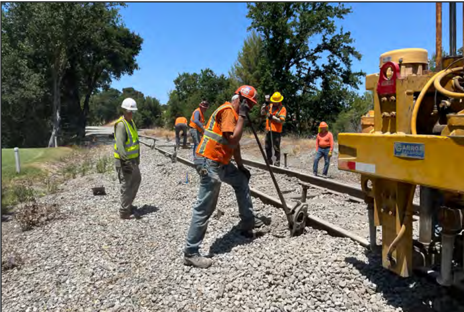
Steve Rusconi removing track jack as tamper advances, June 7, 2025. Mike Pechner photograph
