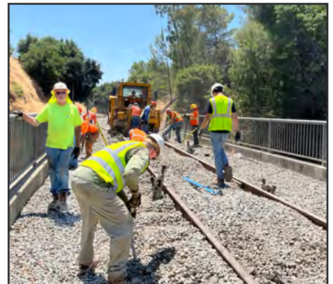
Track jacks positioned to raise the rails ahead of the tamper. Mike Pechner photograph
