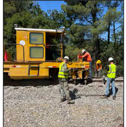
Tamping track approaching Castlewood Bridge, June 7, 2025. Mike Pechner photograph
