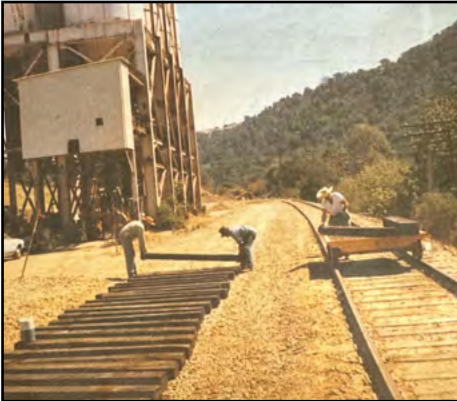
Dexter Day photograph Tim Flippo and Bones laying out ties for Brightside Siding.
