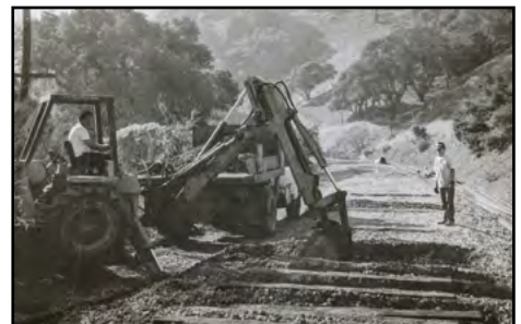
Dexter Day photograph Mark Whitman and Bones Andrews digging out ties at MP 30.5. Nothing was easy.
