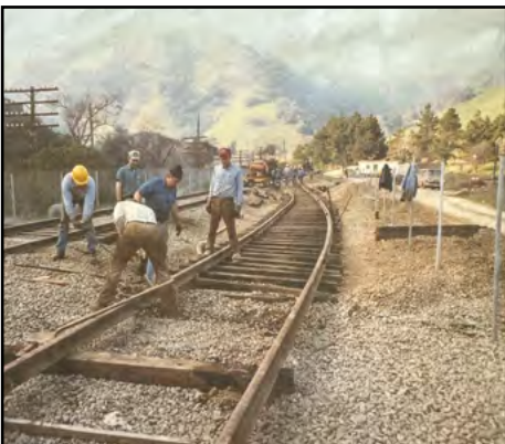
In the beginning, it was to rebuild the railroad. Here is a crew hard at work putting in the passing siding at Brightside.
