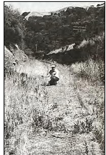
Peter Schulze photograph Castro Point Railway volunteer Dexter Day at the cut East of the Kaiser Killite Plant (Brightside) during Pacific Locomotive Association's mid-1980's inspection of Niles Canyon ROW following abandonment by Southern Pacific a couple of years earlier.
