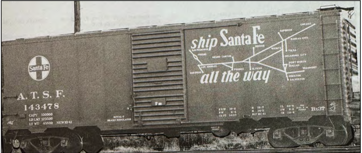
Old picture of BX-37 with B-1 trucks and tac board high on door.
