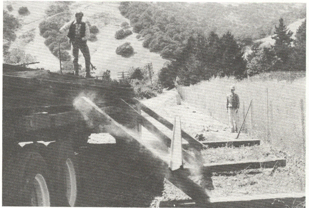
Phil Orth unloading rail at Brightside in June.
