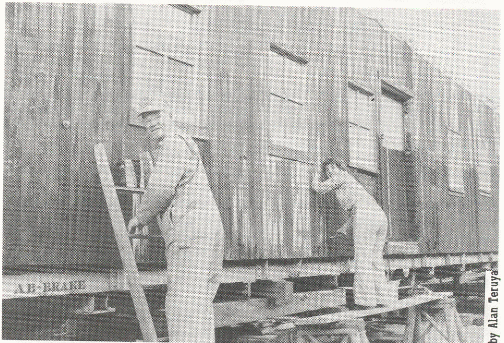
Herb Norleen and Madeline Iverson put a new coat of paint on the NCSRy's new tool car.
