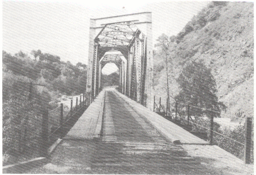
The Rosewerner (or Dresser) Bridge was built in 1906 and crosses Alameda Creek and Highway 84 a mile and a half east of Mission Blvd.
