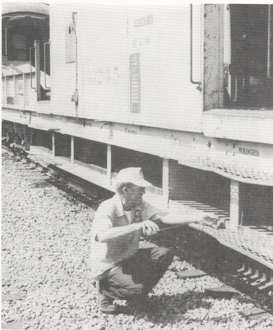
"Bones" Andrews measures the underframe of the AT&SF car at Oakland Army Terminal. This car was converted by AT&SF into a tender for a crane and will be used in Niles Canyon as an open air observation car.
